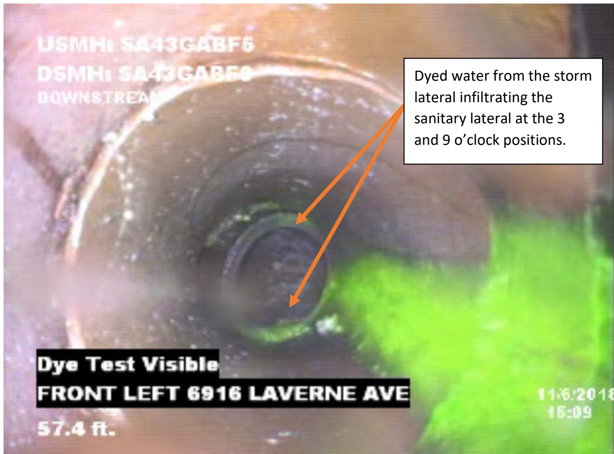
Figure 3-9. Downspout Water Infiltration into Sanitary Lateral
